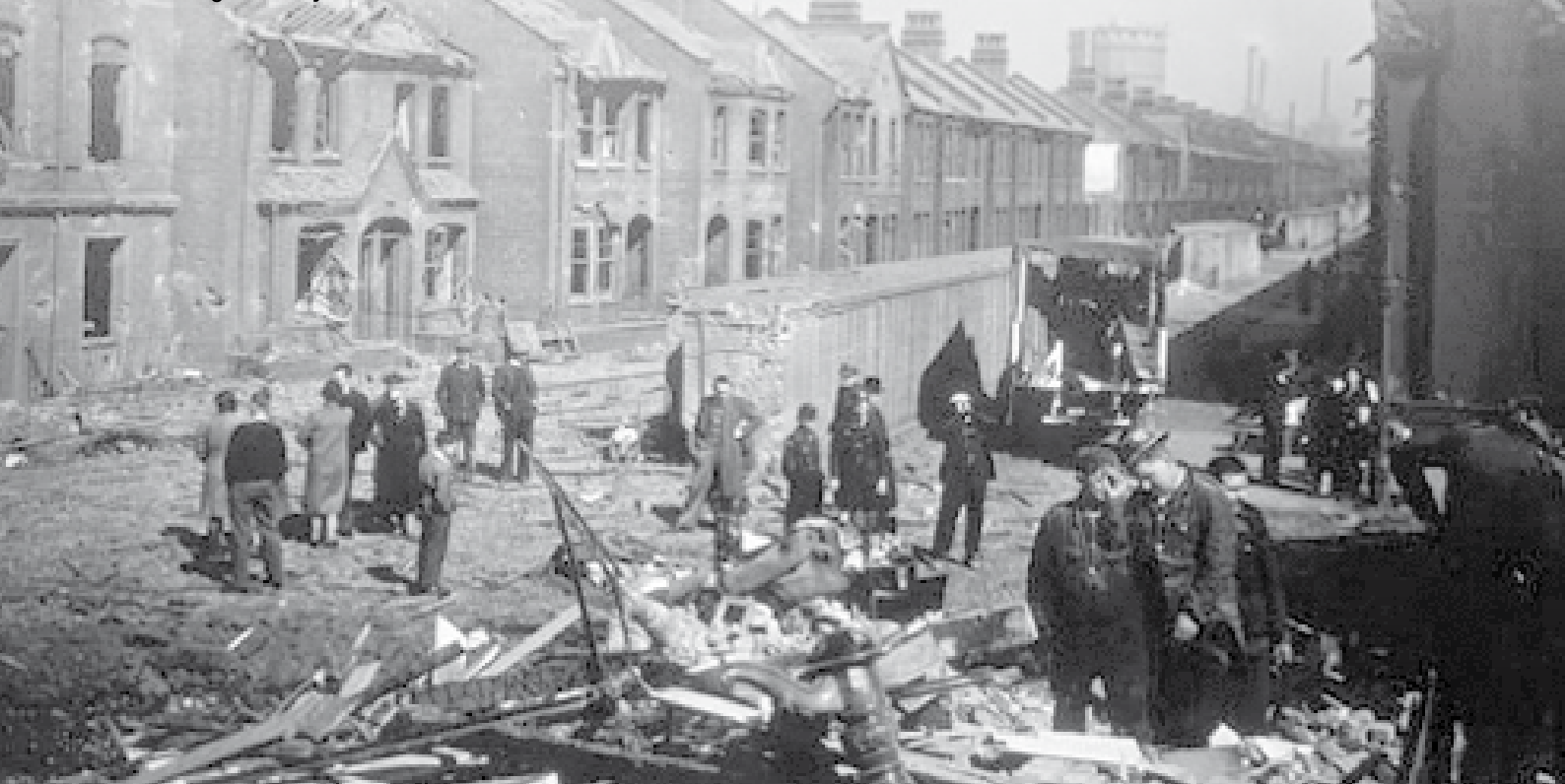
Bomb damage in Tennyson Street
