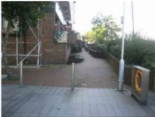
Narrow pathway obstructed by flower beds and low brick walls
