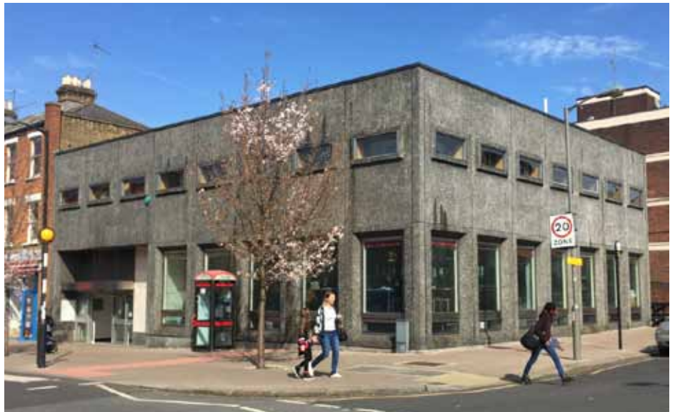
Top: A new library for the 21st century Above: the old building, now being demolished
